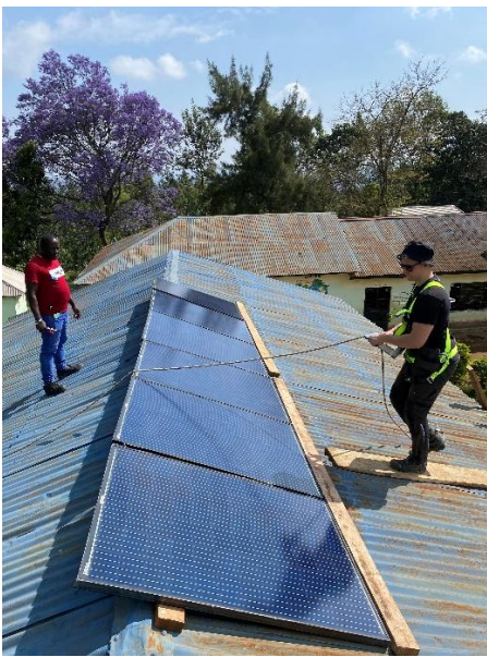
Installation af solcelleanlæg, Nkoanrua Primary School, GLOBUS
